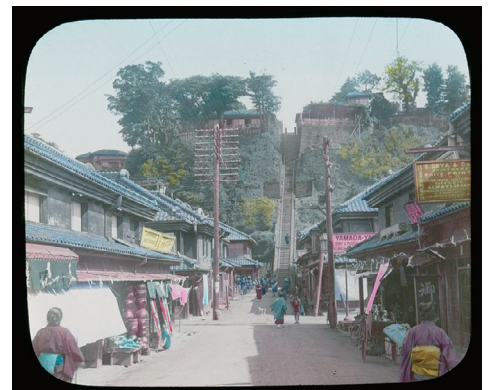
50. 101 Stone Steps at Yokohama (百一段、横浜)
